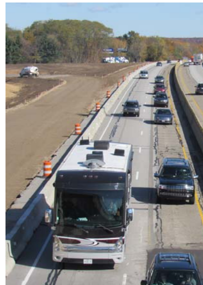
View of I 94 from the Sprinkle Road Bridge.
